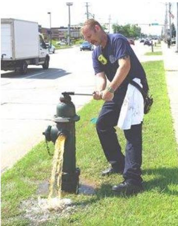
Hydrant flushing started in April, 2023 and were completed at the end of August. SFD inspected and flushed 3,306 hydrants, fifty-two were marked out of service (OOS) for various reasons. The OOS hydrants were forwarded to the Service Department, which will coordinate with Cleveland Water Department to make repairs in 2024.
