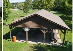
Near Railroad Tracks (#2)
