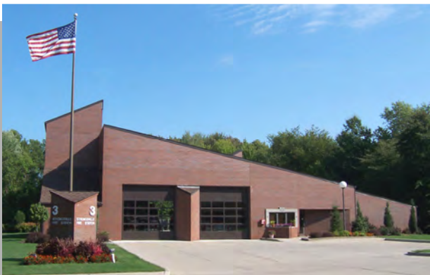
SFD Station 3 22000 Albion Road Dedicated 1980
