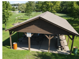
Near Railroad Tracks
